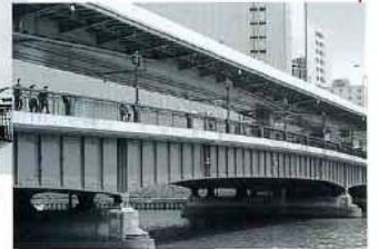
The bridge today. The New Temma Bridge was constructed right above the Temma Bridge in 1970. Those two bridge are called "Kasane bashi" (two-story deck bridge) since then.
