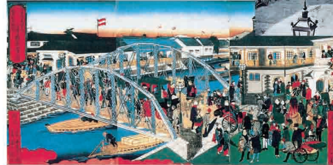
"Picture of the Shinsai Bridge" by Sadanobu Hasegawa II (Kobe City Museum) The bridge is now preserved in Tsurumi Ryokuchi Park.
