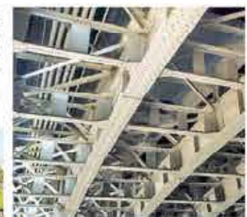
Underside of Tenjin Bridge
