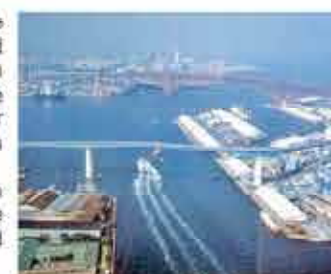
Naniwa-Ohashi Bridge and Minato-Ohashi Bridge, Bay Area
