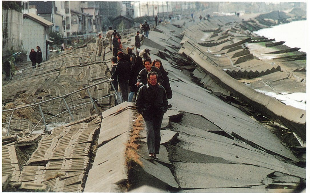
▲ The embankment at the mouth of the Yodo River; collapsed portion 1800 m (January 17, 1995)
