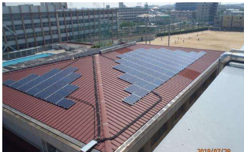
市設建築物の屋根の貸し出しによる太陽光パネル設置促進 (長吉西中学校) Promoting solar panel installation by renting out roofs of municipal buildings (Nagayoshi West J.H.S.)
