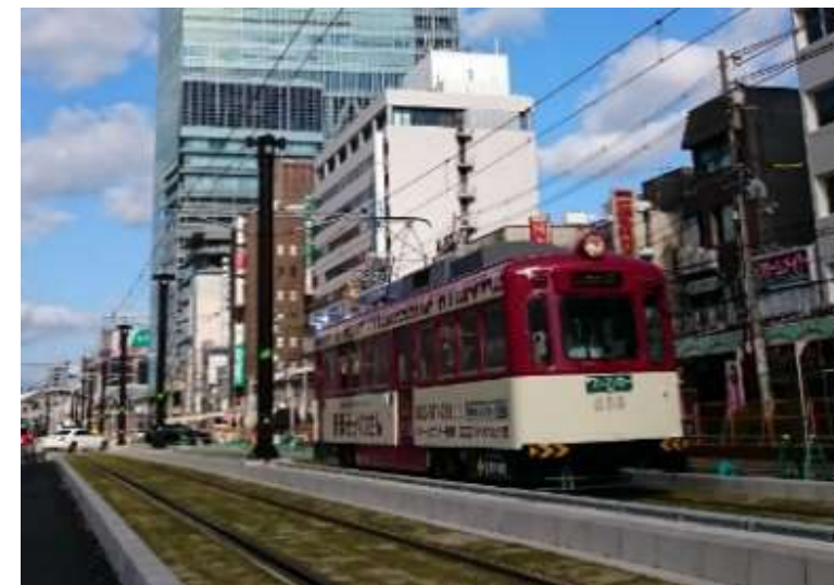
軌道敷緑化 (阪堺電車) Greening of track bed (Hankai Tramway)
