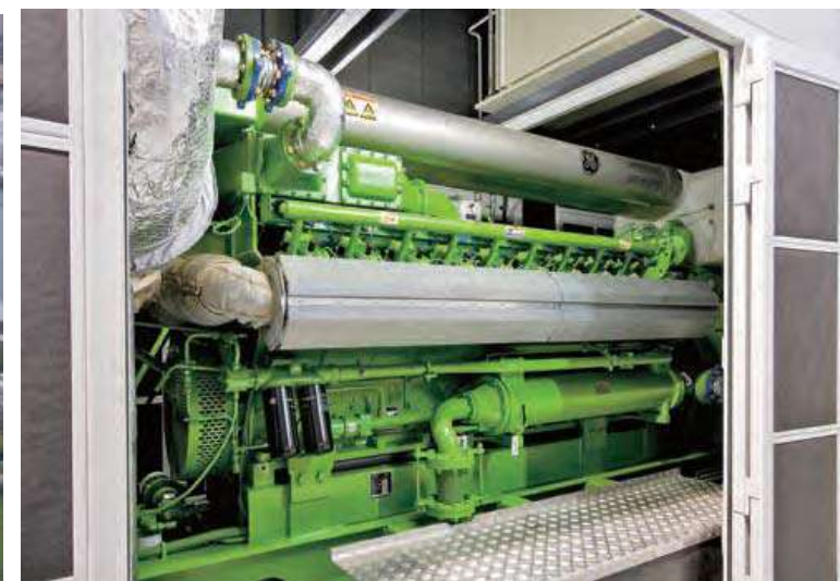
津守下水処理場の消化ガス発電 PFI generator at Tsumori Wastewater Treatment Plant
