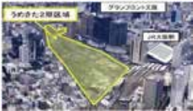
■ "Umekita Second Development" where new urban development is proceeding
