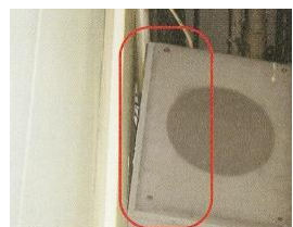
拡声装置の取付不良❖ 3
