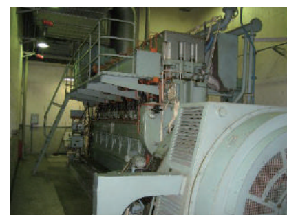
Private power generation equipment for facility operation (Tatsumi water distribution plant)
