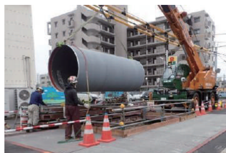
Earthquake-proofing construction of pipelines (Tatsumi first water pipe)
