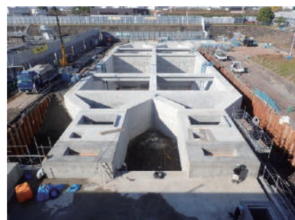
Earthquake-proofing construction of water intake facilities (Kuzuha water intake plant)
