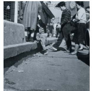
Collapsed road due to land subsidence
