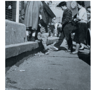
Collapsed road due to land subsidence
