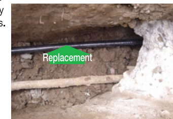
Replacement of lead water supply pipes
