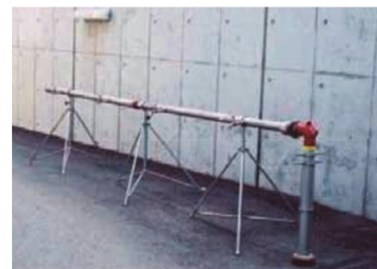
Material for emergency water supply (temporary water taps)
