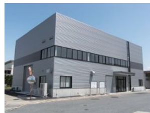
Optimum cutting-edge technology testing facilities
