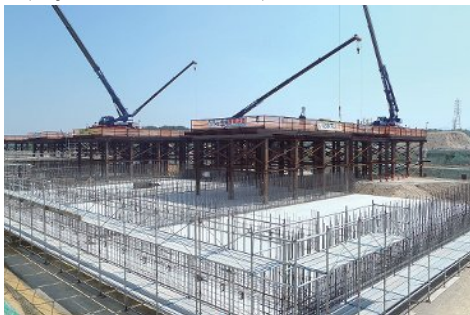
■ Figure: Earthquake-proofing of Toyono Purification Plant (coagulation and sedimentation basin)
