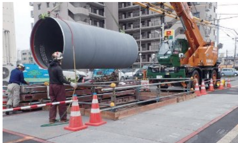
Figure: Updating of large-diameter pipeline (PIP method)
