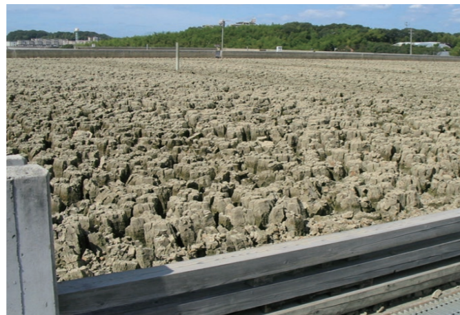
Solar drying system (Toyono Purification Plant)
