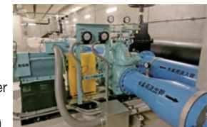
Hydroelectric power generation system at Sakishima Distribution Plant
