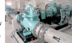
Hydroelectric power generation system at Izuo Distribution Plant
