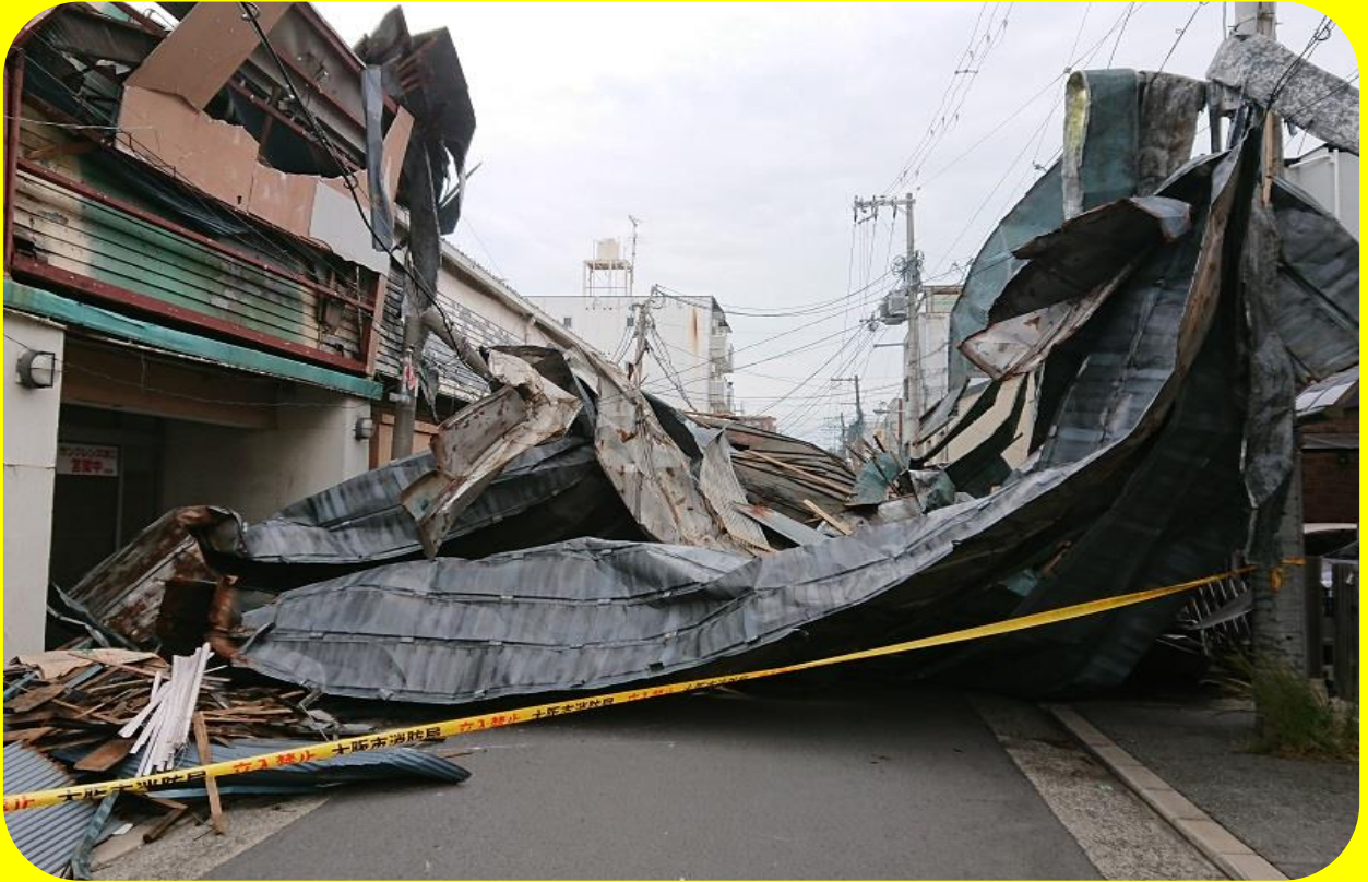
Photo of Osaka City area damaged by Typhoon Jebi in 2018.
