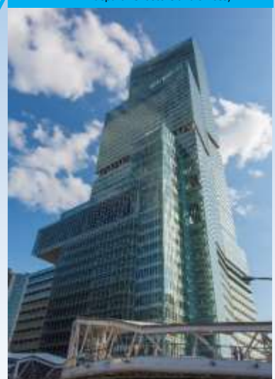
ABENO HARUKAS (Observation deck, hotel, museum, department store and offices)
