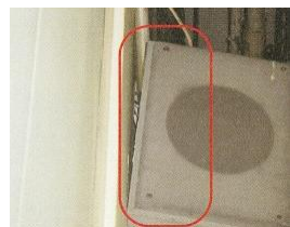
拡声装置の取付不良❖ 3
